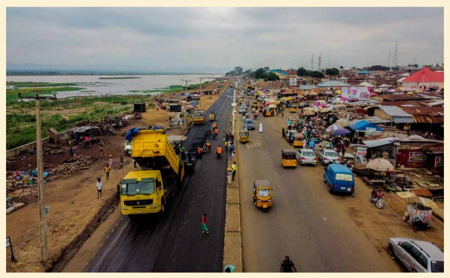
Reconstruction and Asphalt Overlay of Natako - Paparanda Square Dual carriage way
